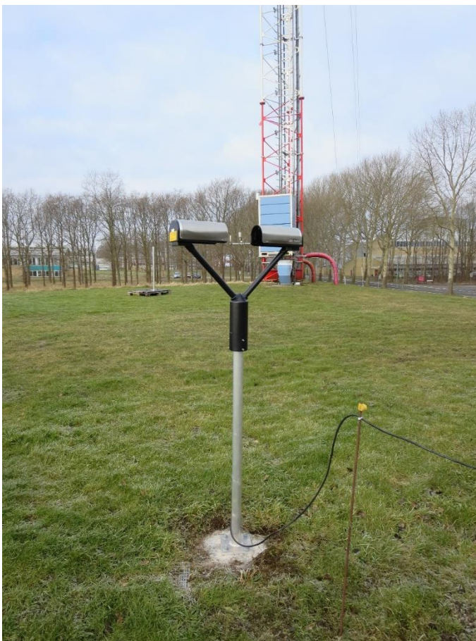
Figure 3: Disdrometer installation at DTU Risø campus next to the tall meteorological mast (RMM)
