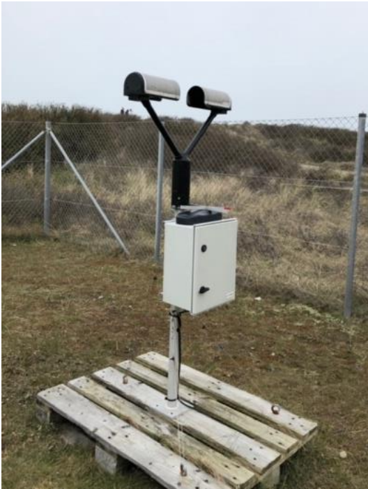
Figure 7: Disdrometer installation in Thyborøn - DTH
